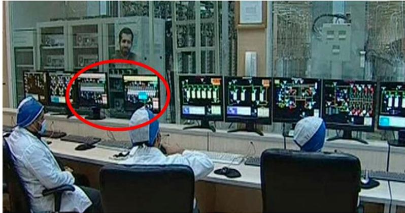
The control room of the above-ground Pilot Fuel Enrichment Plant (PFEP) as of February 2012, with operators sitting in front of SCADA screens. The two displays highlighted in red run the monitoring application for the Cascade Protection System that is discussed in-depth in this document.
