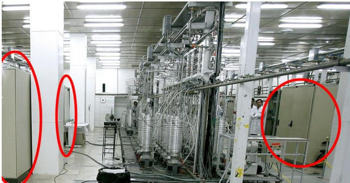
Location of control system cabinets in the above-ground Pilot Fuel Enrichment Plant (PFEP). Although it cannot be seen in the picture, the Siemens S7-417 and S7-315 controllers compromised in the attack are almost definitely located inside these cabinets – which will likely have been accessed directly by the control system engineers who unwittingly infected the controllers with Stuxnet.
