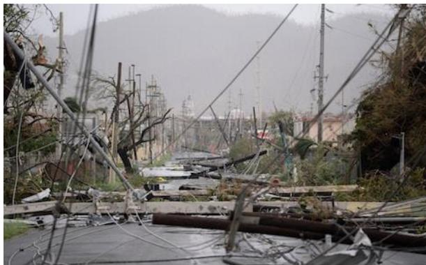
*Figure 2. Image of downed power and communication lines caused by Hurricane Maria.*
