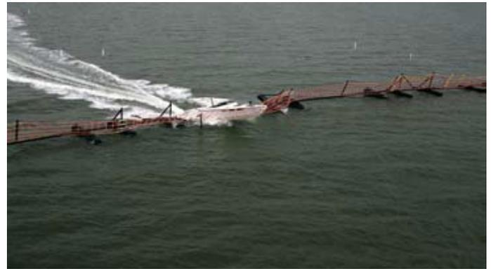
Figure 3: Net Boat Barrier
